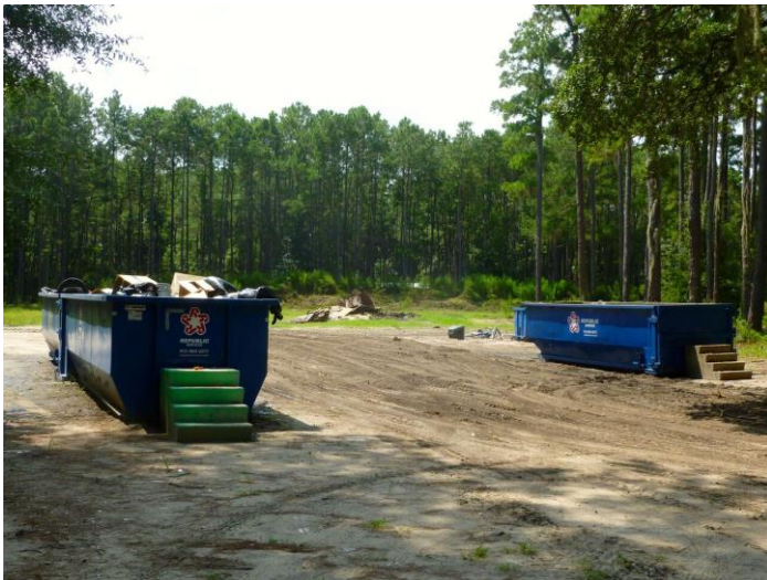
Current Convenience Center: Unpaved, No Fence
